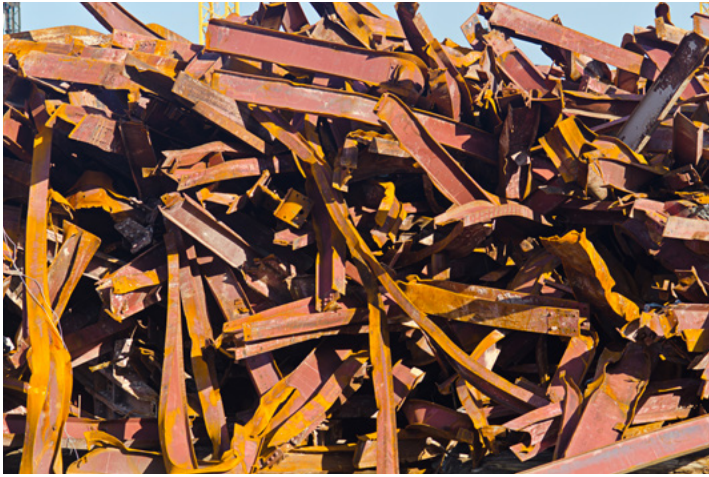
Debris from the demolition of the Grand Palace Hotel/Claiborne Towers building, New Orleans.
