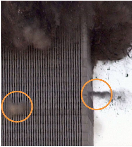
High-velocity bursts of debris, or “squibs,” were ejected from point-like sources in WTC 1 and WTC 2, as many as 20 to 30 stories below the collapse front.
