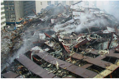
WTC 7's steel structure was dismembered and deposited into a compact debris pile.
