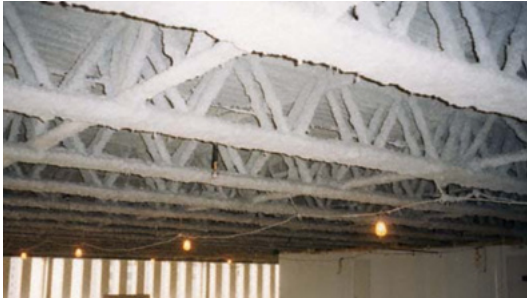
A photograph of WTC trusses with fireproofing.
