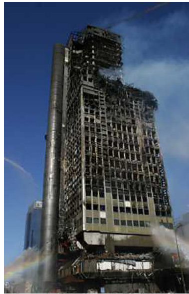
The Windsor Tower after having burned for almost 24 hours.
