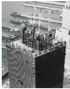
WTC 1 during construction.
